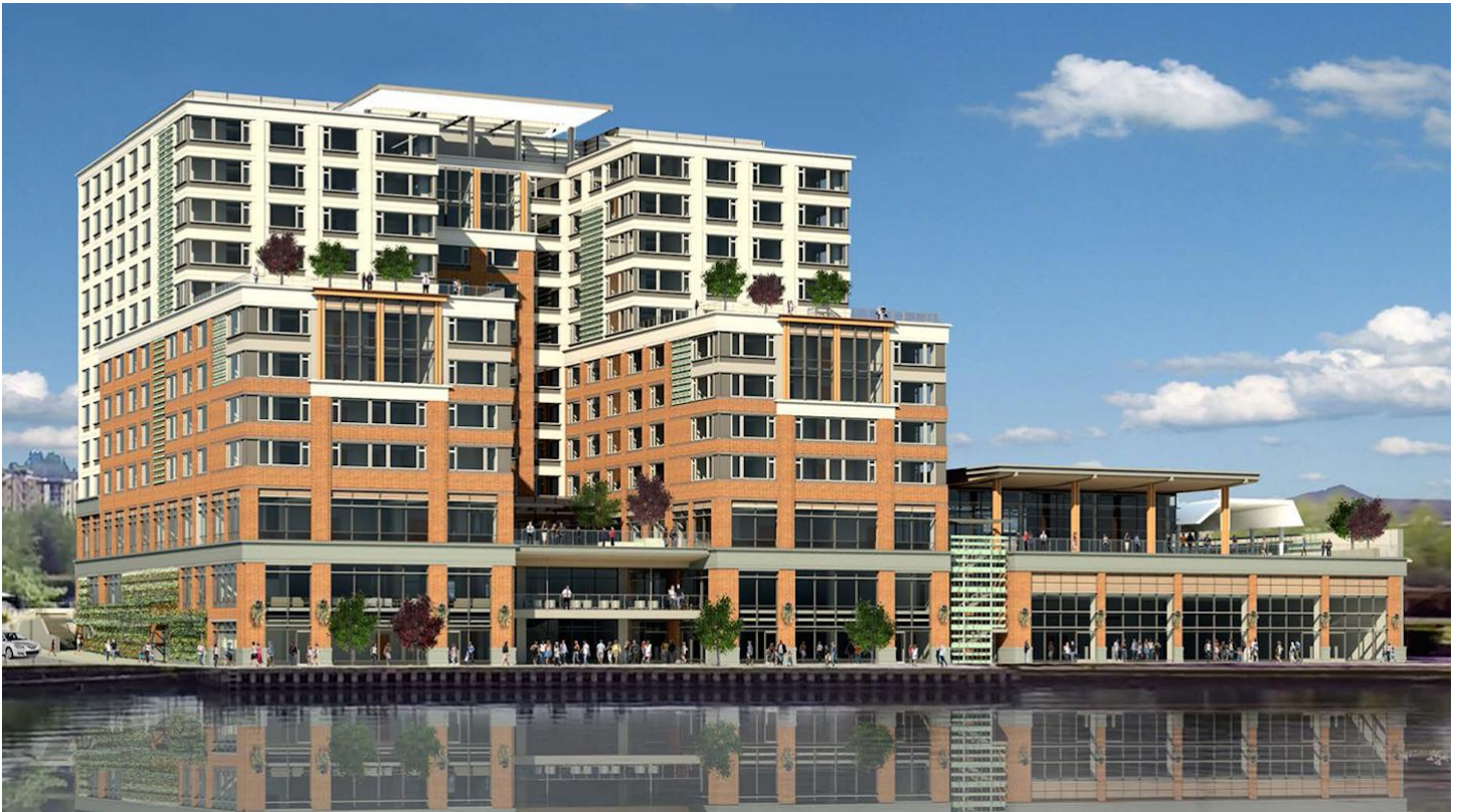
The 12-story 4-star Hotel at Southport is now under construction SW from our venue and immediately east of the Boeing 737 hangar. It won't be complete for the COW until 2017, and Boells has already booked his room.
