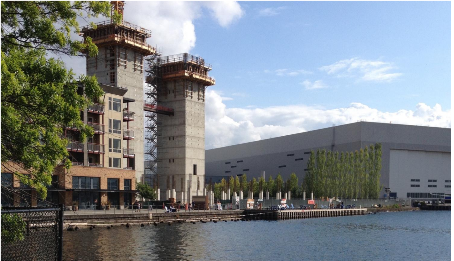
Hotel at Southport under construction between the 7-story condos on the left and the Boeing 737 hangar. Bob Wells photo.
